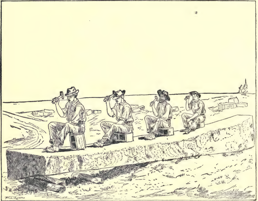
FIG. 7.—DRILLING HOLES FOR SPLITTING STONE WITH PLUG AND FEATHERS.
